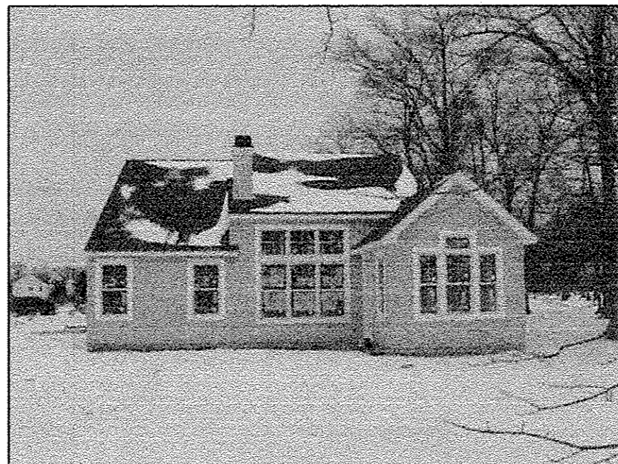
UNIT #21 REAR VIEW
