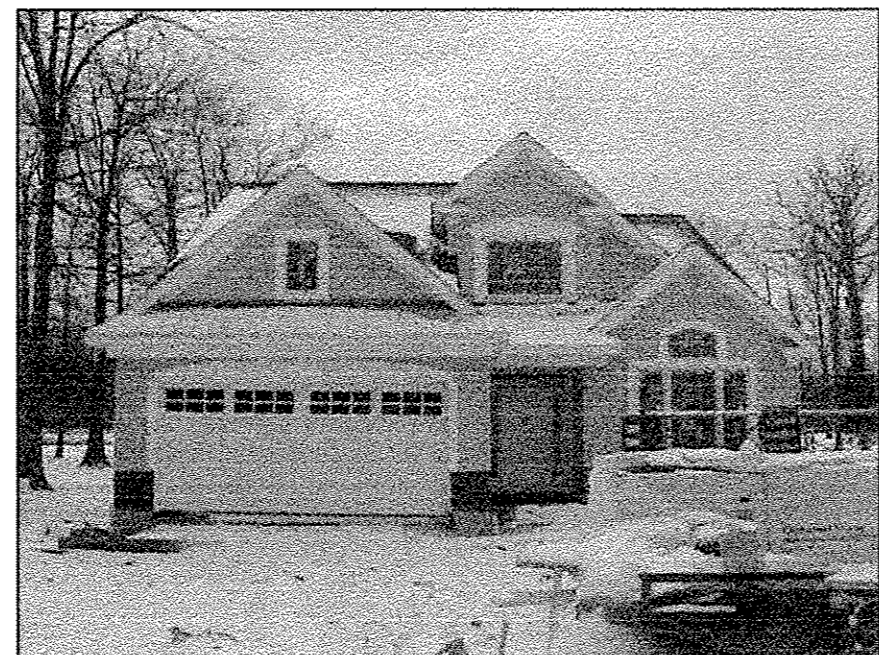
UNIT #21 FRONT VIEW
