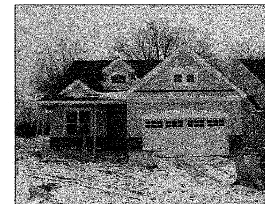
UNIT #17 FRONT VIEW
