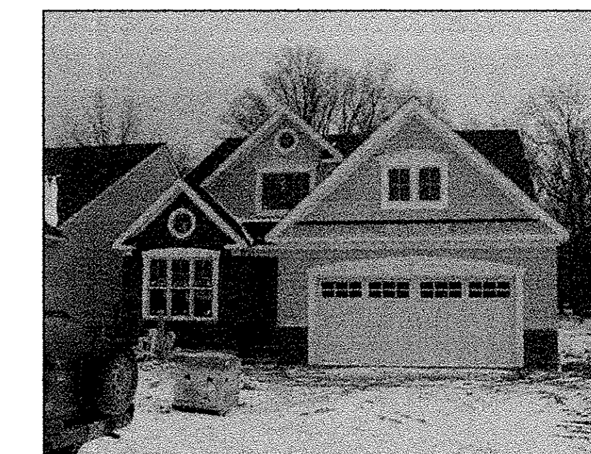
UNIT #18 FRONT VIEW
