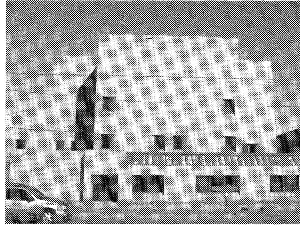
EXISTING CONDITIONS (SOUTH)
