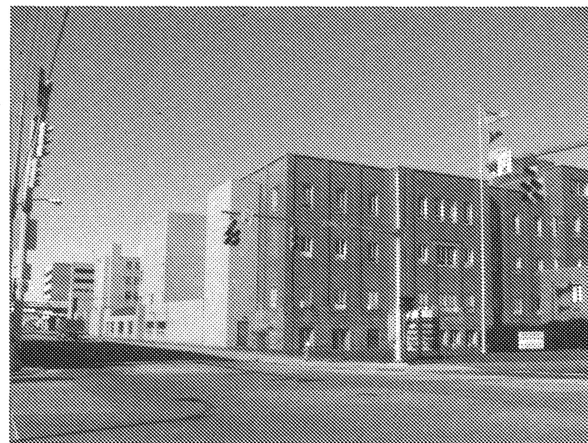
EXISTING CONDITIONS (SOUTHEAST)
