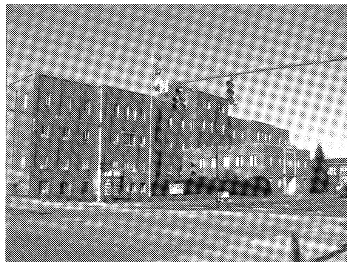
EXISTING CONDITIONS (SOUTHEAST)
