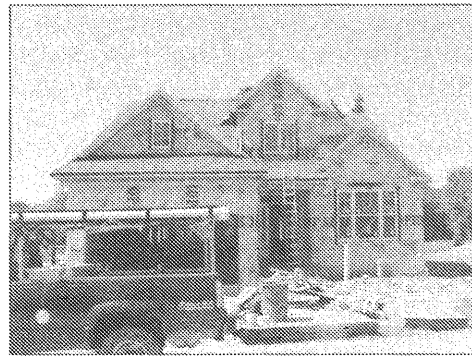
UNIT 10 FRONT VIEW
