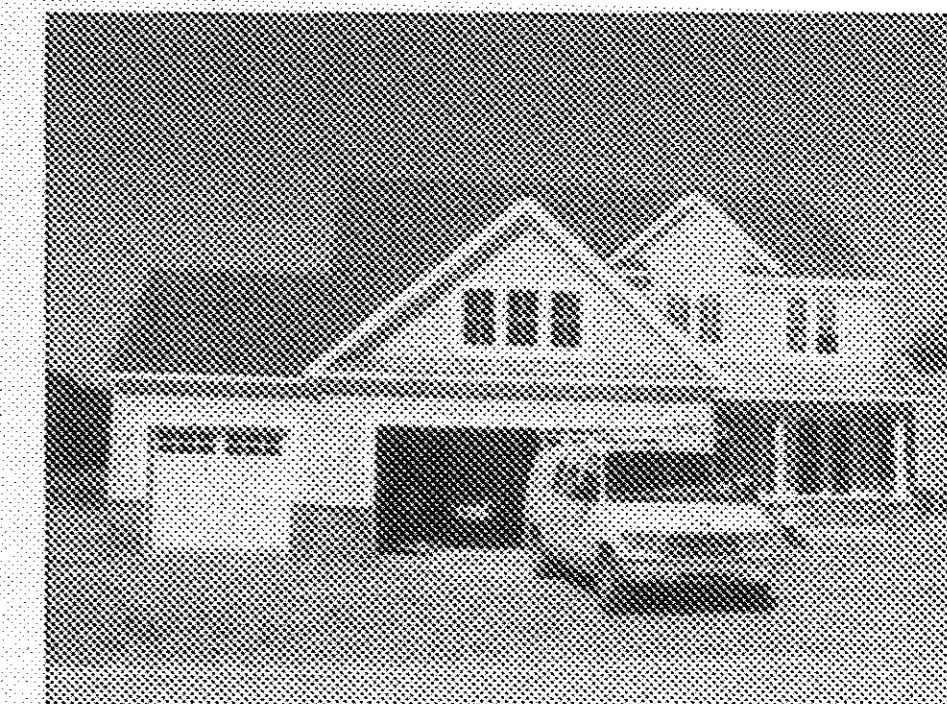
UNIT 8 FRONT VIEW
