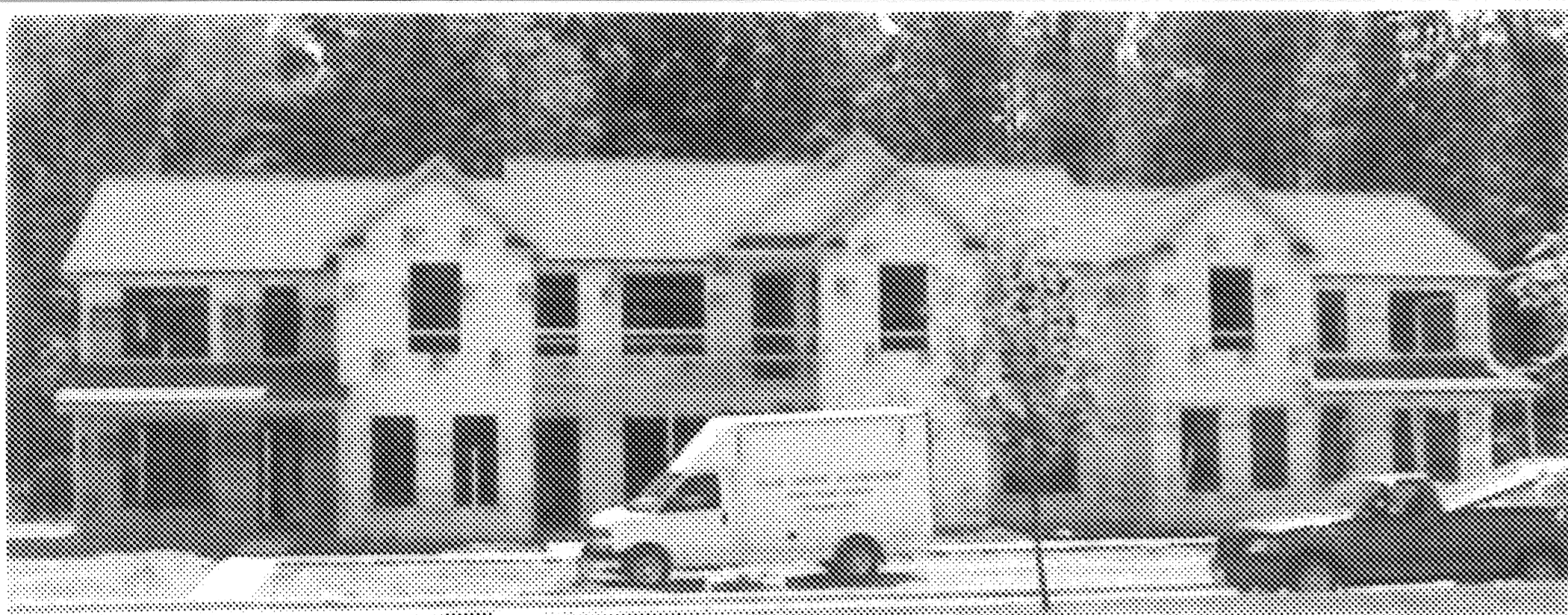
BUILDING 31, NORTH SIDE
