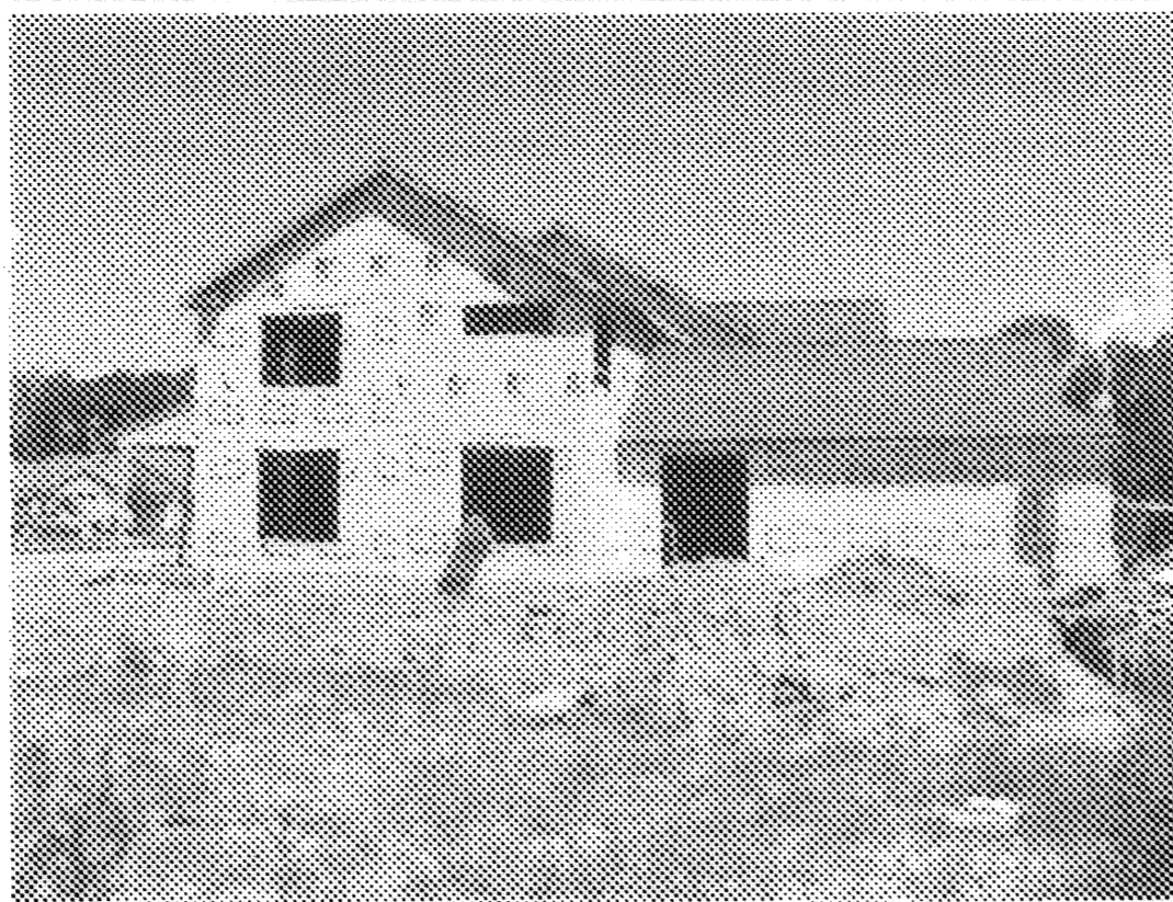
BUILDING 31, WEST SIDE
