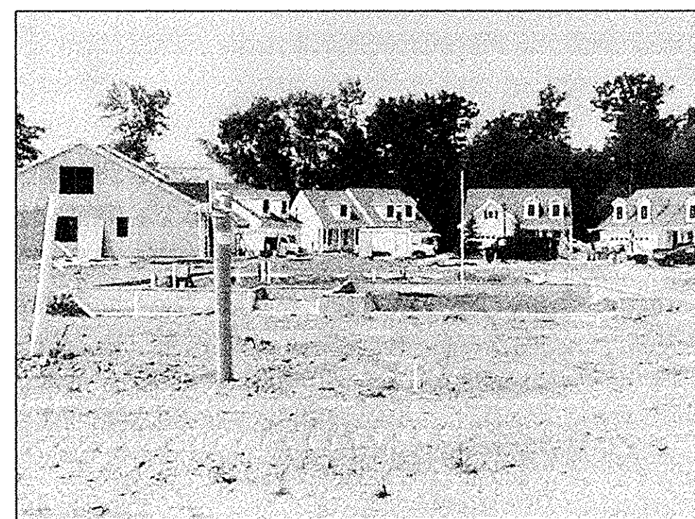
UNIT No. 22 FOUNDATION
