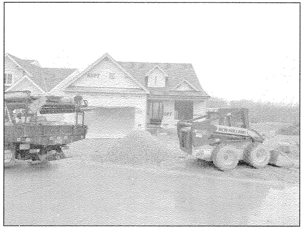
UNIT #51 FRONT VIEW
