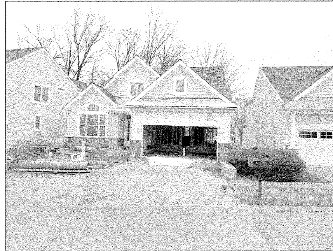
UNIT #49 FRONT VIEW
