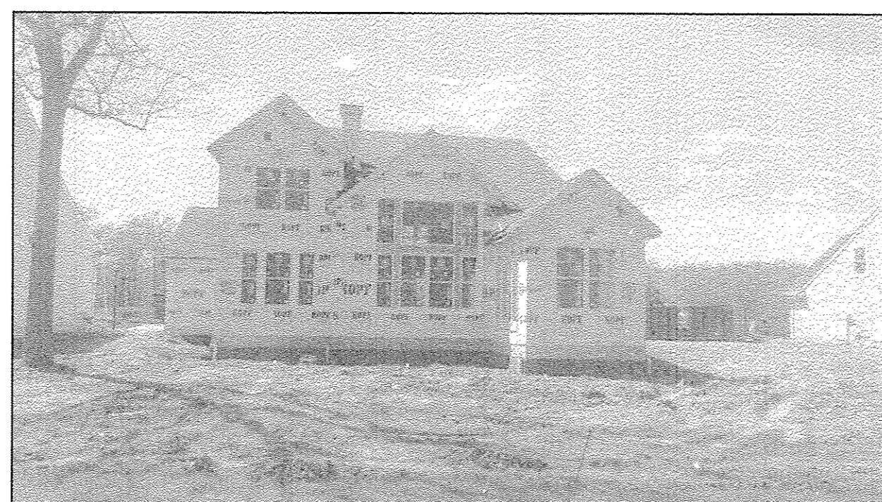
UNIT #46 REAR VIEW
