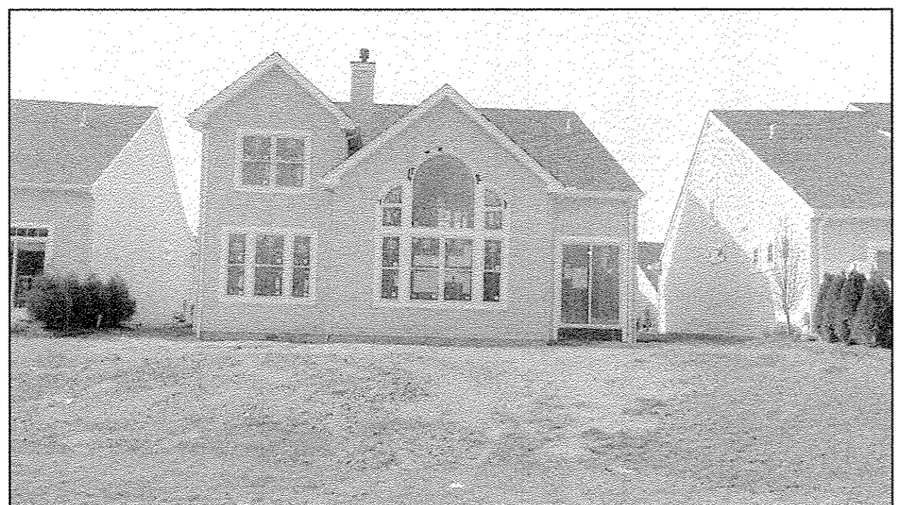
UNIT #42 REAR VIEW
