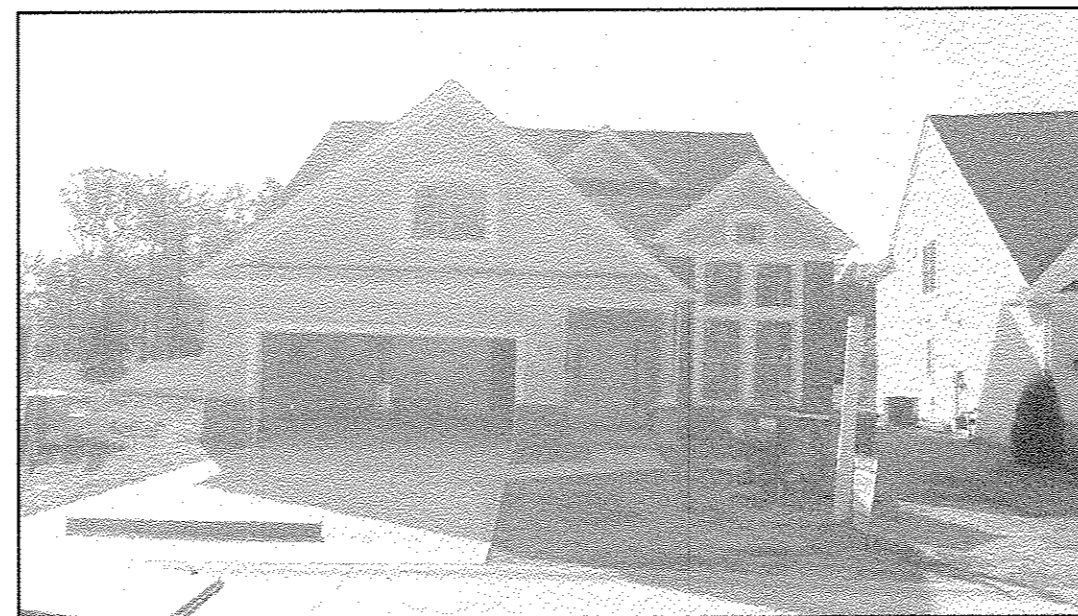
UNIT #38 FRONT VIEW
