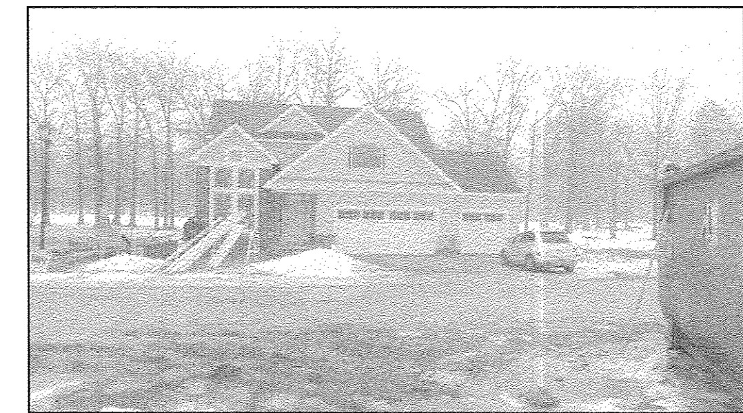
UNIT #32 FRONT VIEW
