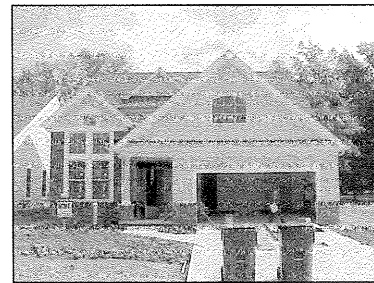
UNIT #28 FRONT VIEW
