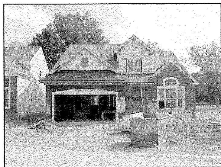
UNIT #27 FRONT VIEW
