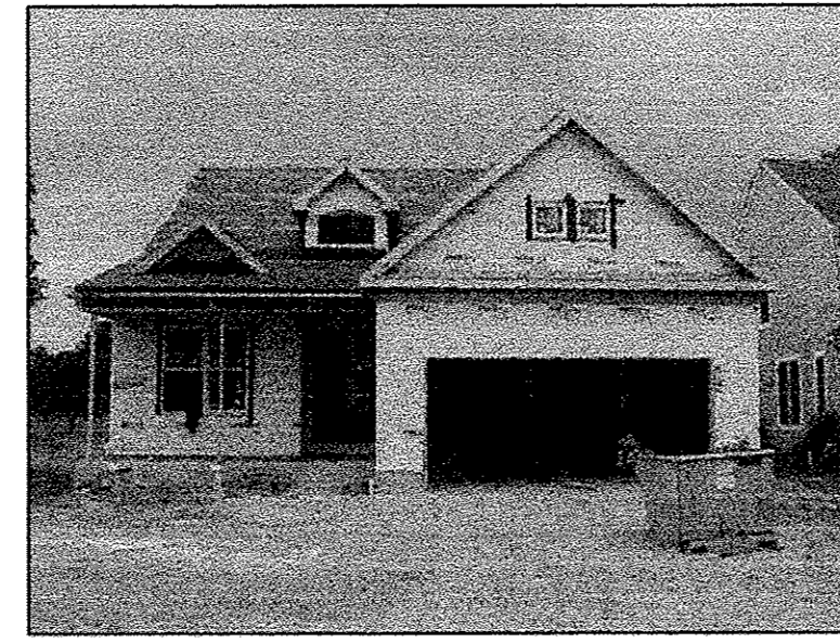
UNIT #24 FRONT VIEW
