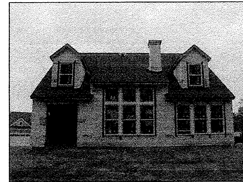
UNIT #23 REAR VIEW
