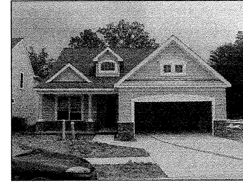
UNIT #25 FRONT VIEW
